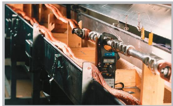
***Crimping is a System Technology. This means that it is the combination of a choosen terminal or connector and a matching crimp tool, all determined by the specific conductor that will result in the desired connection properties.***
