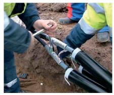
Use a socket wrench to tighten the screws. It is also possible to use an impact wrench.
